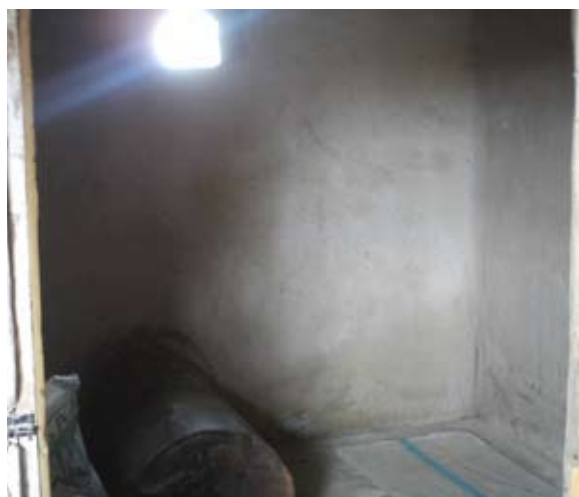
Hole to allow spent air to be vented during drying.
